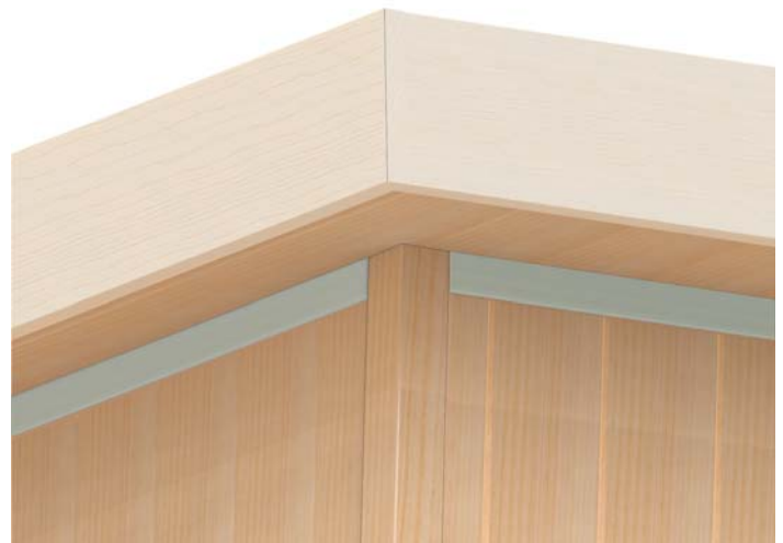
Figure 28. Installing Exterior Cove Trim
